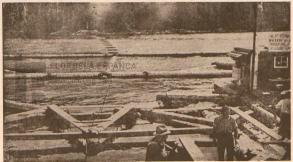
ON A FLOATING SALMON TRAP IN SOUTHEASTERN ALASKA The wire poundnet is suspended beneath the log framework and held down by weights. The wire net «lead» (marked by floats) extends to shore from center of trap. The light and owner's sign (seen at right) are required by law.
